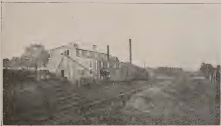
(29) Custom Mill, Kentucky Fluorspar Co., at Marion.
